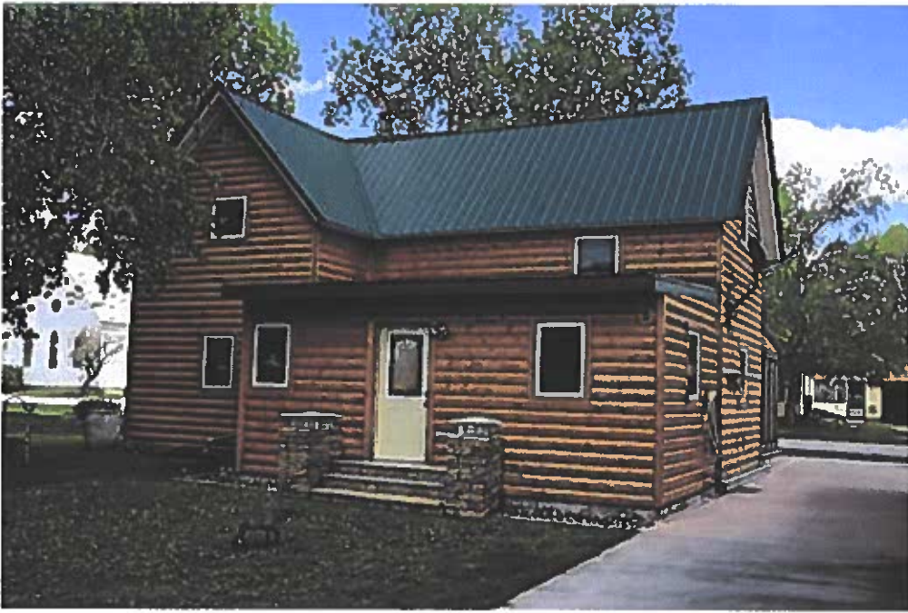
Sample of Roofing
